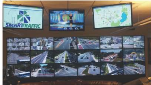
Traffic monitoring cameras collect traffic information as part of the Traffic Management System and send it to the City of Gainesville Traffic Management Center.
