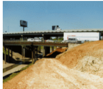
New trail construction
