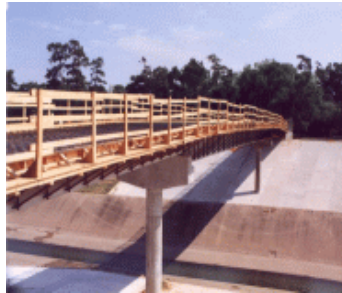
Pedestrian bicycle bridge
