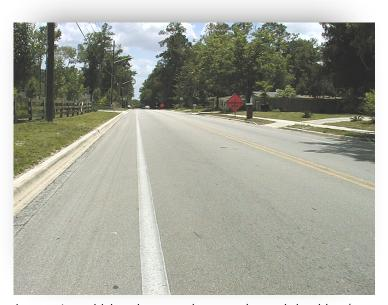
Low motor vehicle volume roadways and paved shoulders/bike lanes provide good bicycling conditions.
