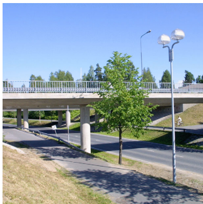
Separated path with 5' distance 3' elevation at suburban arterial road. Paths provided on each side of street with bicycle designated overpass. Oulu, Finland
