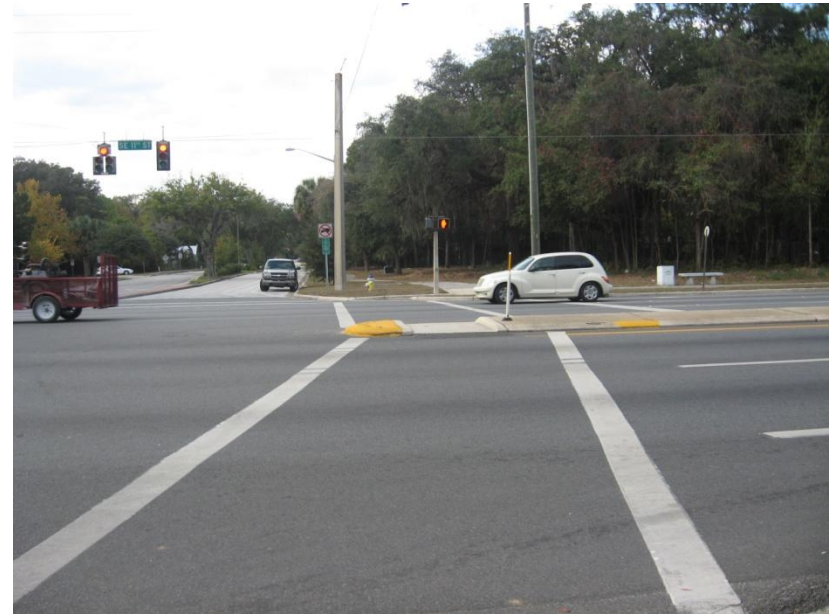
Figure 8.1.1: View west at SE 11 th St crosswalk. Lack of striping and a long crossing distance are present.
