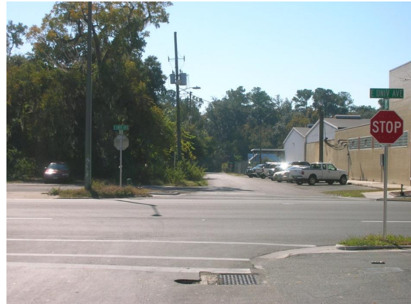
Figure 8.4.2: View south at intersection at SE 10 th Avenue and University Avenue. Improper intersection alignment and lack of sidewalks and bike lanes create a harsh environment for non-motorized users.
