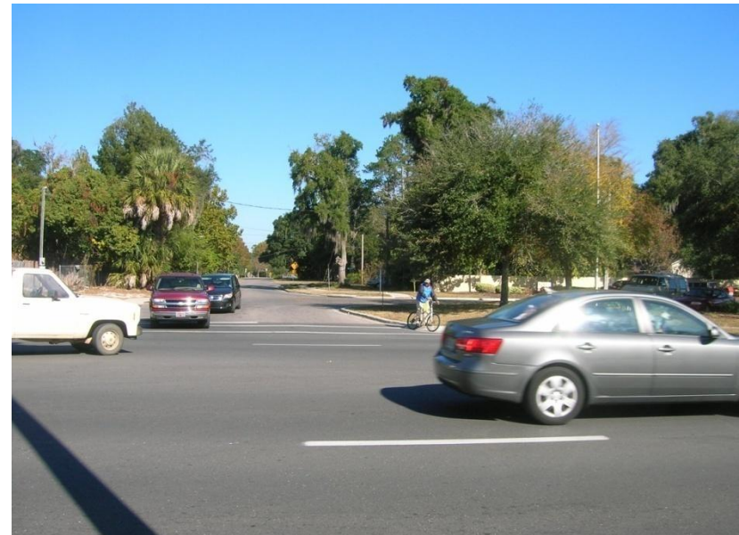
Figure 8.4.1: View north at intersection of SE 10 th Avenue and University Avenue. No pedestrian refuge and high speed traffic deters non-motorized use.
