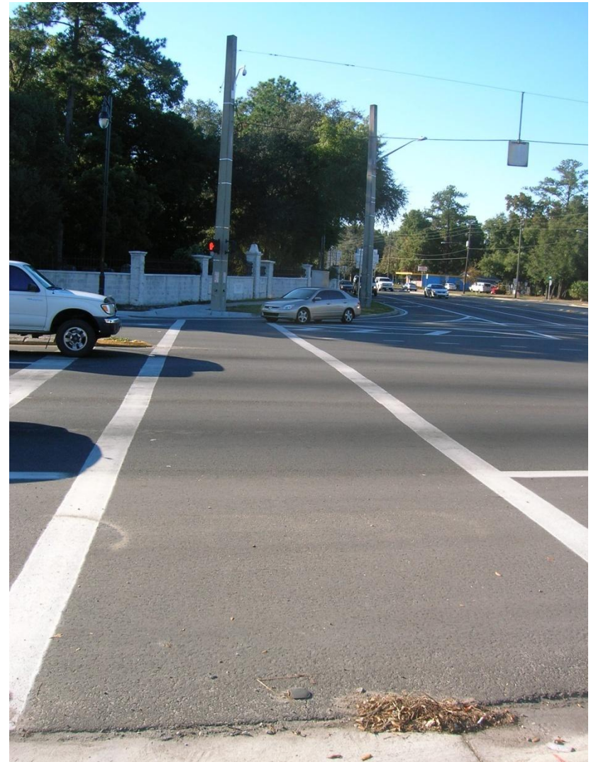
Figure 8.6.2: View south at the intersection of Waldo Road and University Avenue. Pedestrians and cyclists crossing north are unable to see the traffic signal and are vulnerable to right turning vehicles (see figure 8.6.5 below).
