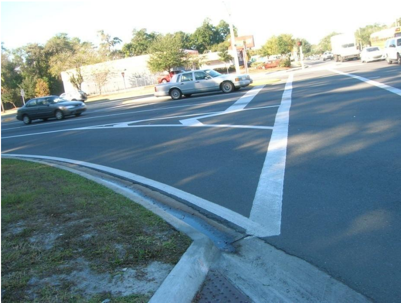
Figure 8.6.3: View west at the intersection of Waldo Road and University Avenue. Lack of striping and road geometries that cater to the motorist create a dangerous situation for the non-motorist (see figure 8.6.4 below).
