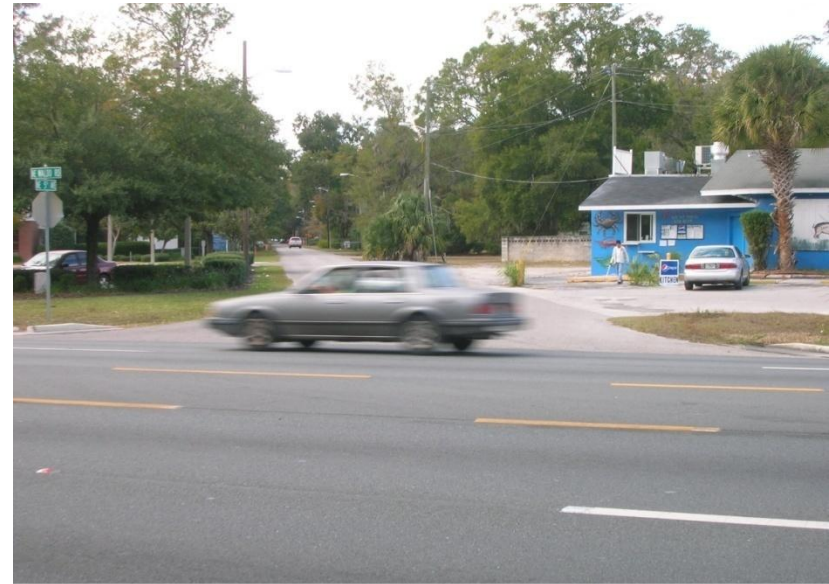
Figure 8.2.1: View west at intersection of NE 5 th Avenue and Waldo Road. No pedestrian refuge and high speed traffic deters non-motorized use.
