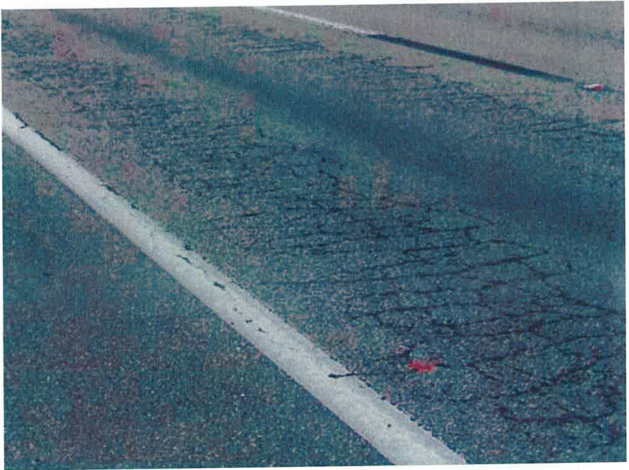
FIGURE 10. CLASS III CRACKING
