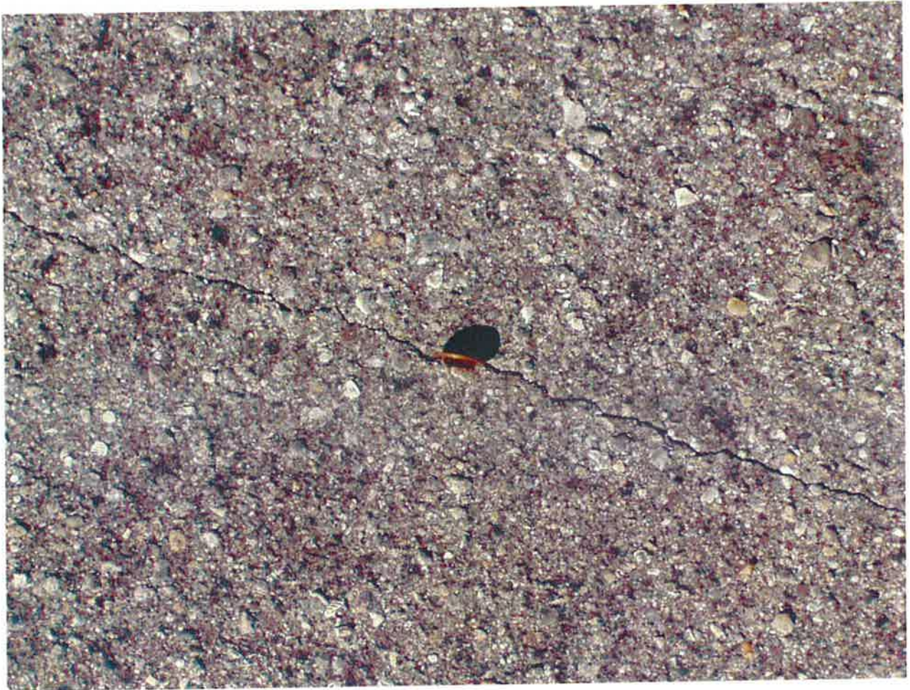
FIGURE 8. CLASS IB CRACKING
