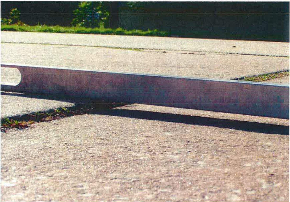
FIGURE 9. FAULTING
