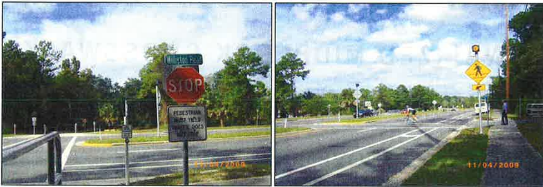
Figure 1: Flashing Signalized Crosswalk on Williston Road in Gainesville, FL
