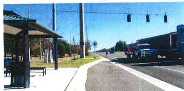
The two photos above are from the same roadway and illustrate an example of a high volume roadway that balances the needs of freight traffic, transit, and pedestrians and bicyclists of varying abilities. The corridor includes a shared use path, bicycle lanes, bus pull-outs, bus shelters with benches, and other amenities. Location: US 98, Polk County, FL. Source: KAI
