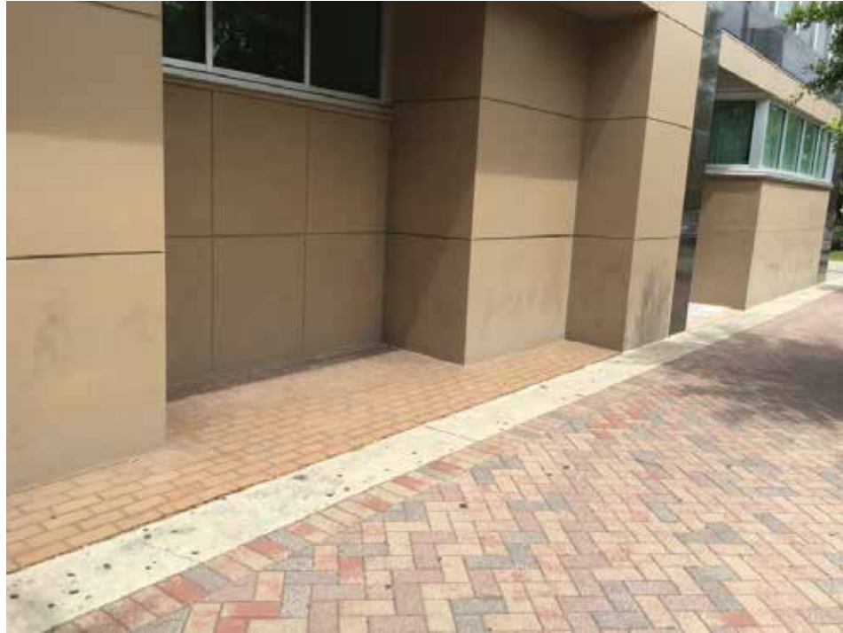
Figure 29 Photo looking east to building opening area next to RTS stop located on westbound SR 26 at NW 1st Street
