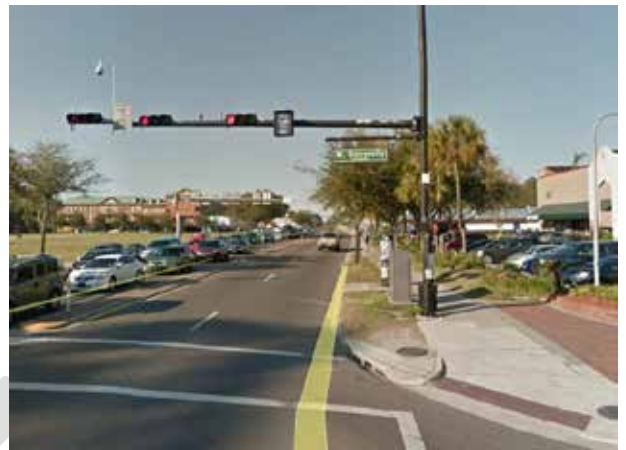
Figure 12 No RIGHT ON RED Blank Out Sign at SR 26 and 13th Street
