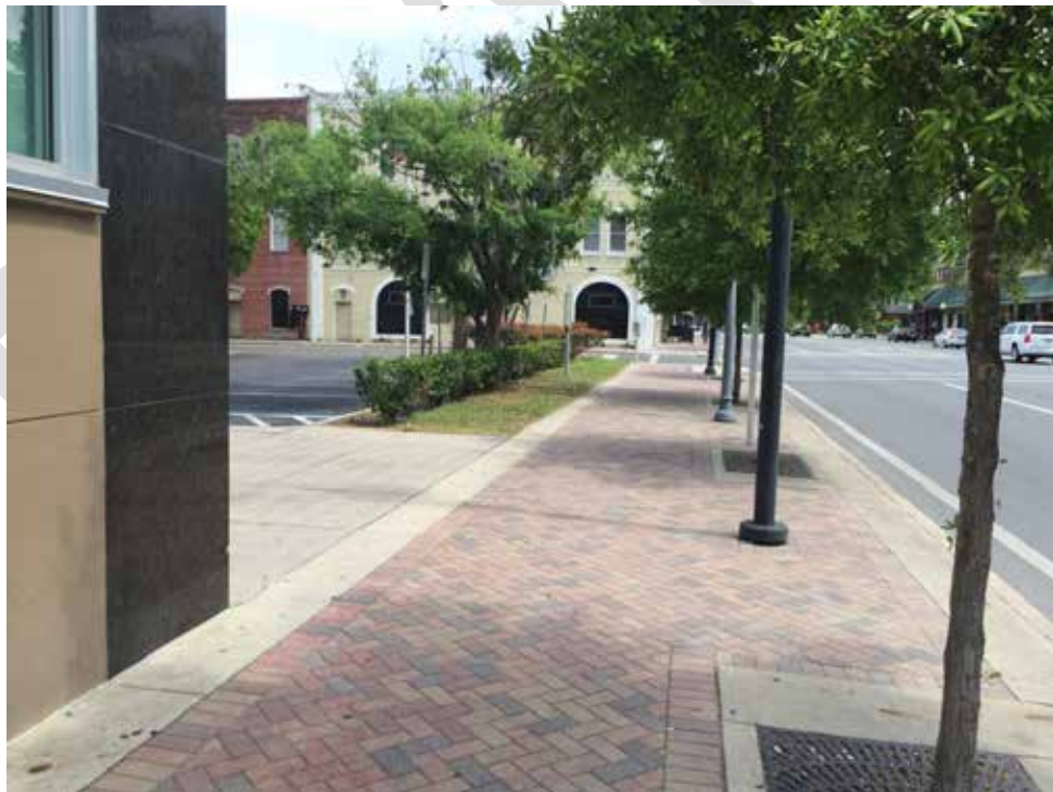
Figure 30 Photo looking east parking lot area next to RTS stop located on westbound SR 26 at NW 1st Street
