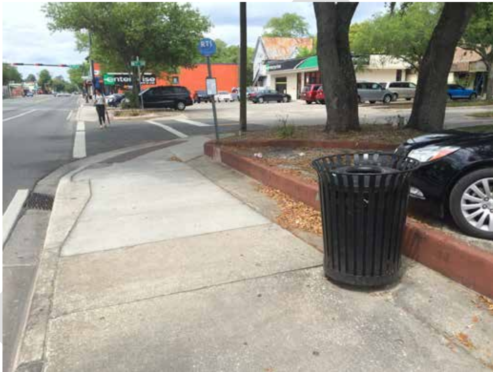
Figure 35 Photo looking west from RTS stop located on westbound SR 26 at NW 7th Terrace
