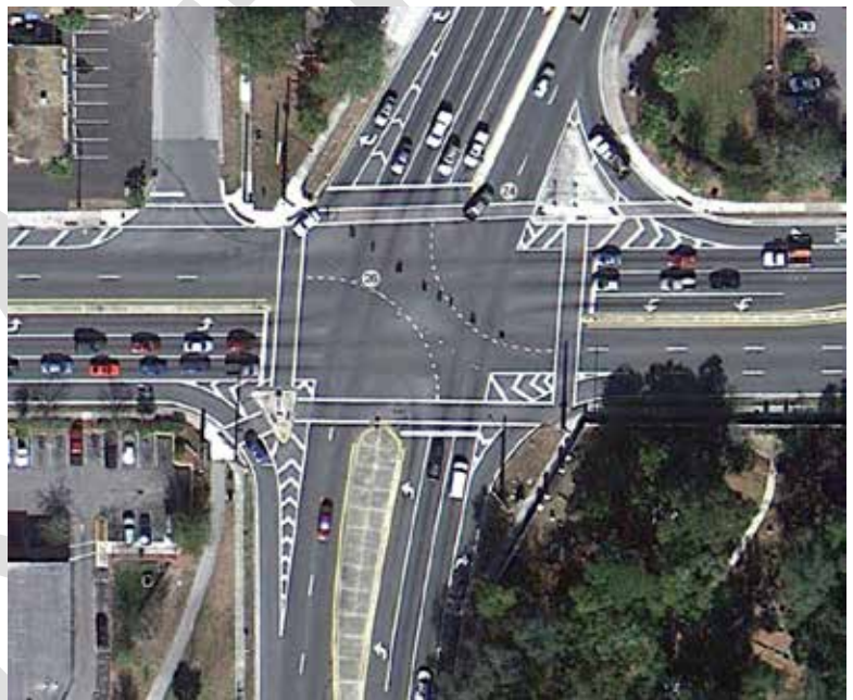
Figure 1 - SR 26 and Waldo Road, Existing Conditions
