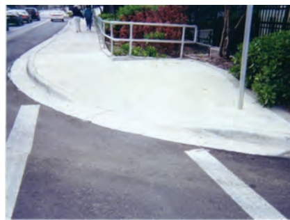
Bad – Missing Detectable Warning
