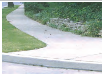
Bad – Missing Curb Ramp
