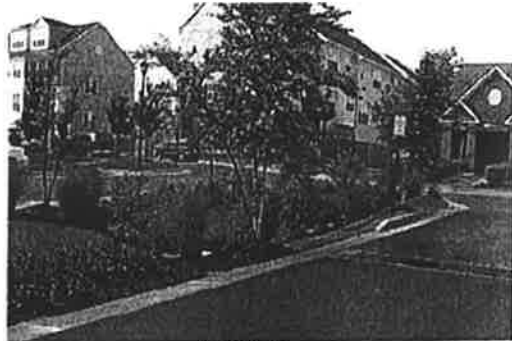
BIORETENTION AREAS (PICTURED ABOVE) ARE ONE EXAMPLE OF A LOW IMPACT DEVELOPMENT (LID) TECHNIQUE
